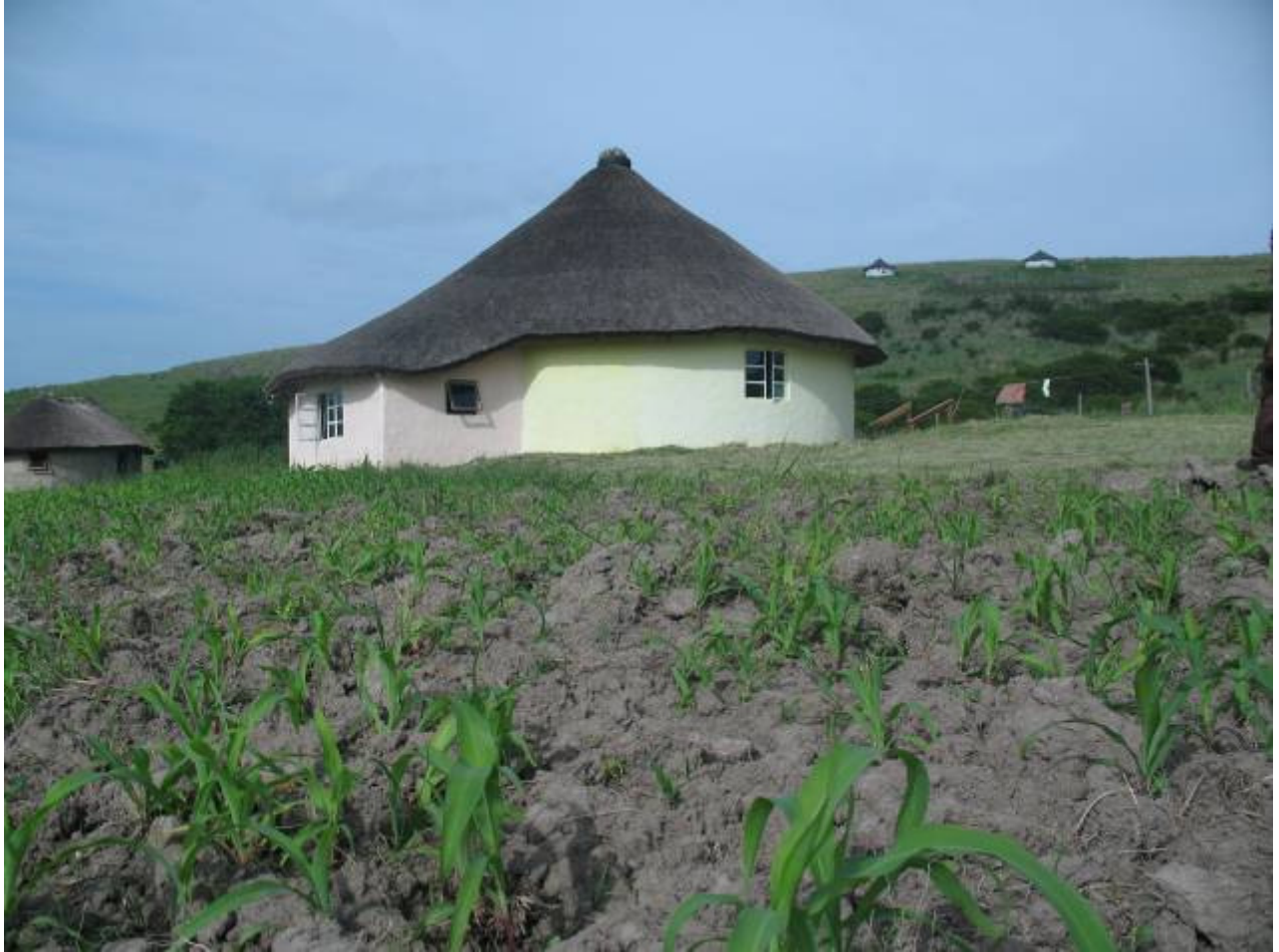
The now limed kitchen/dining/launch rondavel with new mill field in front and bathrooms/toilets in the background.
