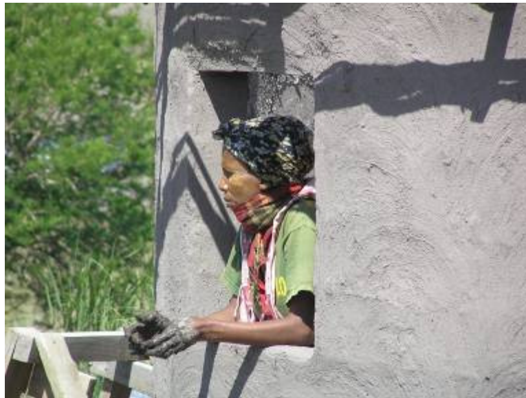
Mamlungu with her hands full of 'plaster'- made out of mud and water. She is taking a break from 'plastering' the new guest cottage.
