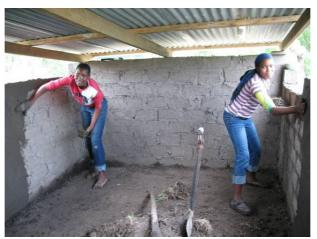
PLASTERING THE GOATSTABLE. THE WHOLE BUILDING, EXCEPT THE CORRIGATED IRON ROOF, IS MADE FROM NATURAL MATERIALS SUCH AS MUD AND FRESH COWDUNG.
